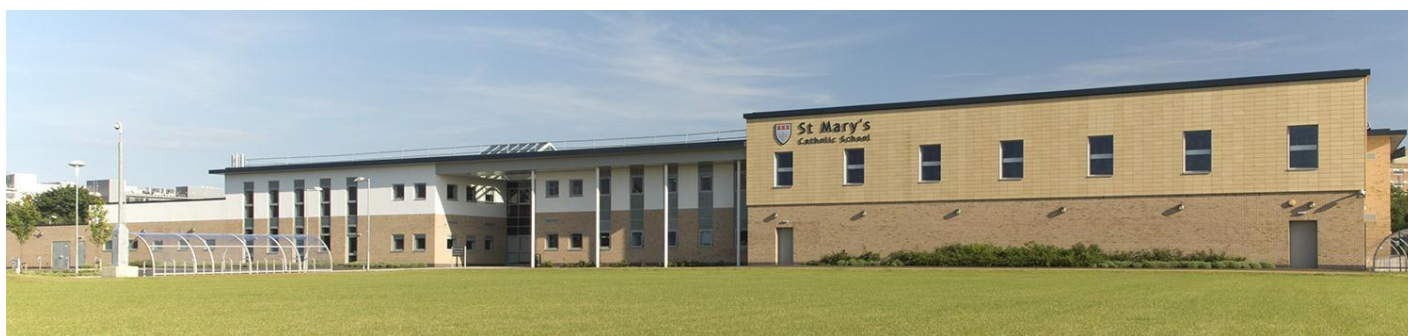
The school – front view
